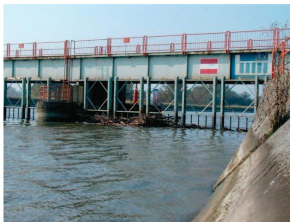
Fig. 6 Probe protection pipe on the bank— clogging of coarse rack
